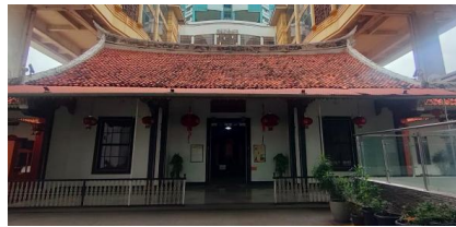
Figure 6 Main Entrance and Main Door from Front and Back Side View. (Source: Author, 2024)
