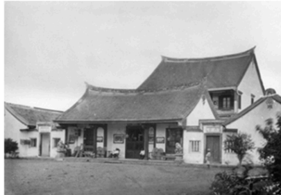
Figure 1 Sin Ming Hui Building, Jalan Gajah Mada No. 188 Jakarta in the 1950s (Source: Kompasiana.com, downloaded December 12, 2023)
