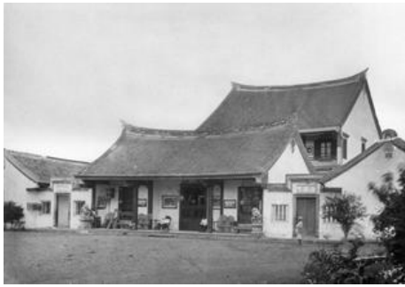
Figure 1 Sin Ming Hui Building, Jalan Gajah Mada No. 188 Jakarta in the 1950s (Source: Kompasiana.com, downloaded December 12, 2023)
