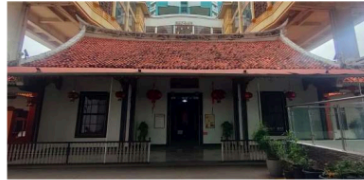
Figure 6 Main Entrance and Main Door from Front and Back Side View. (Source: Author, 2024)
