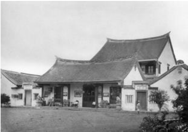
Figure 1 Sin Ming Hui Building, Jalan Gajah Mada No. 188 Jakarta in the 1950s
